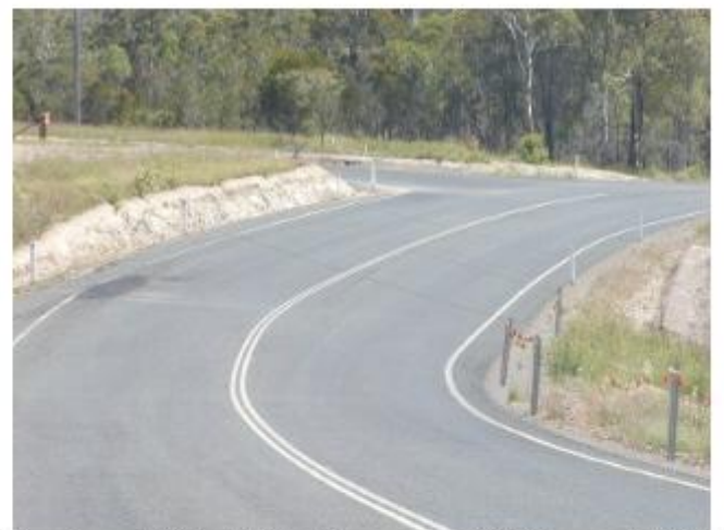
Gowings Hill rd Realignment @ Pipers Ck Rd
