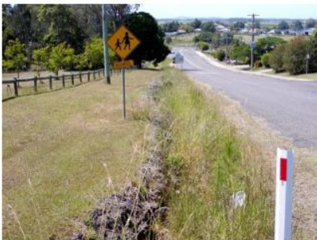
Gt North Road, Frederickton, Road & drainage
