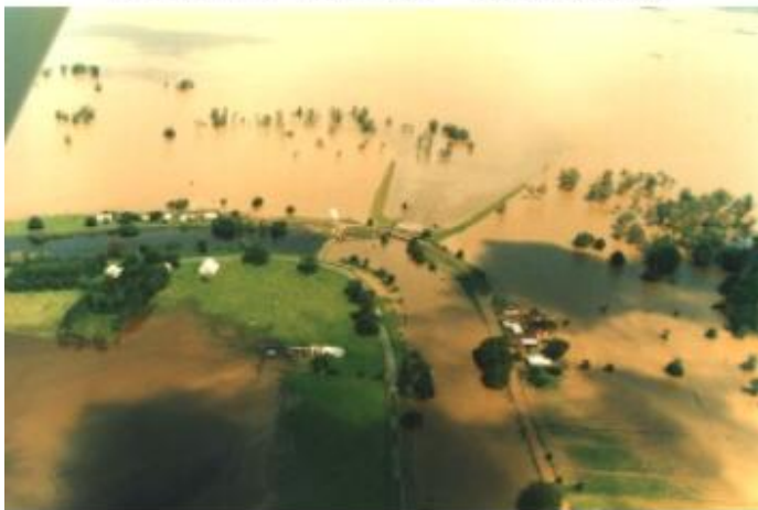
Belmore Flood Control - flooded
