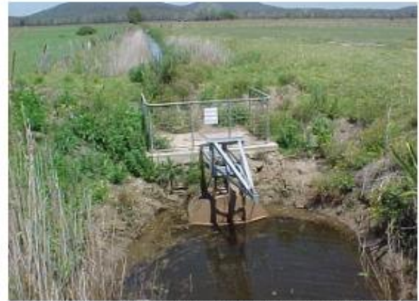
Gate lifting & opening structures
