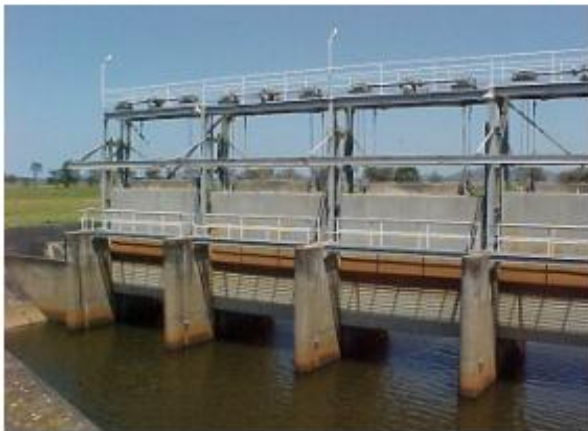
Belmore Flood Gates Refurbished
