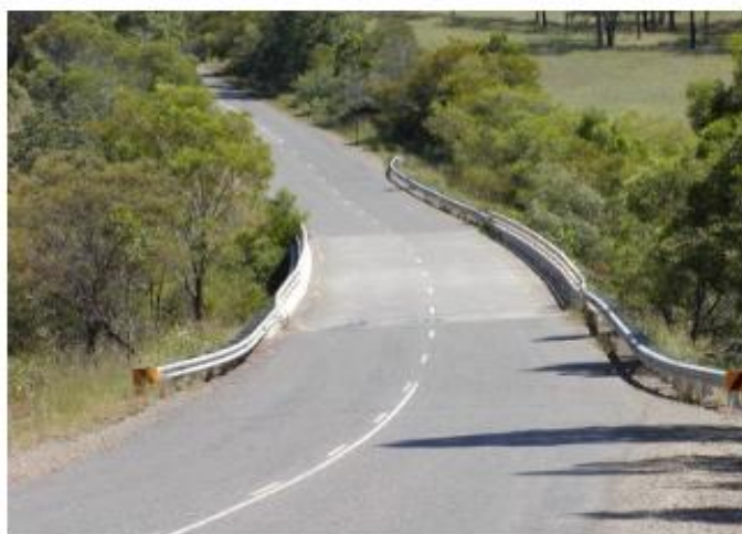
Eureka Creek Bridge
