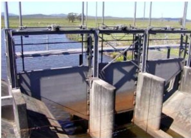
Kinchela Creek Gate Alterations
